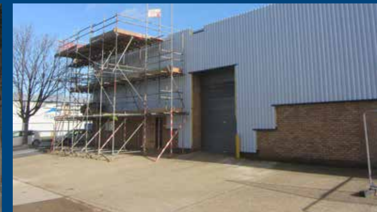
BUILDING MAINTENANCE & REPAIRS
